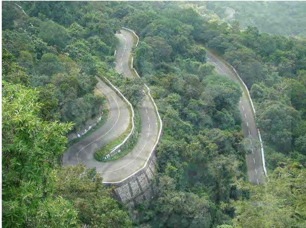
Fig. 2.6.4 Corner Bend and Hair Pin bend
